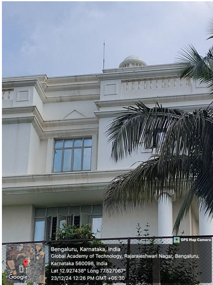
Figure 4-15: Lightning arresters in the college terrace
